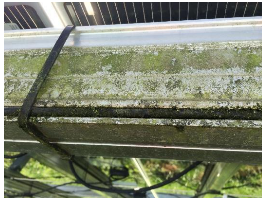
Cable permanently exposed to water
